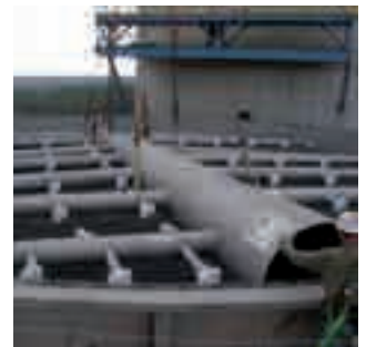
Customized configuration according state-of-art-technologies
